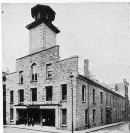
OLD COURT HOUSE
