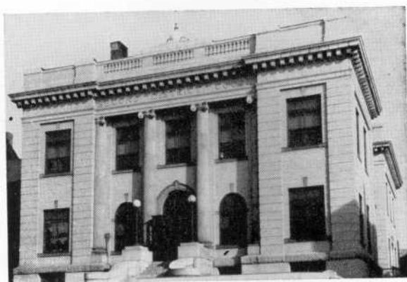
SECOND DISTRICT COURT HOUSE
