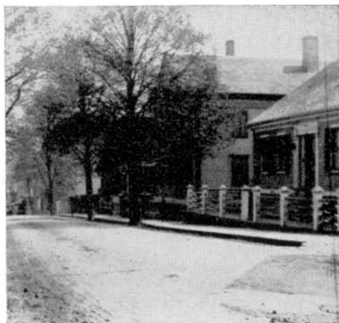
BORDEN RESIDENCE AND DR. KELLY'S COTTAGE ON SECOND STREET
